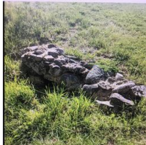
Outfall 37 headwall at southern end of BMP
