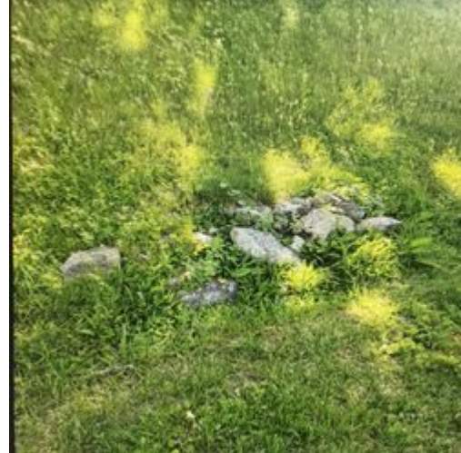
Riprap along eastern side of swale, potentially displaced check dam.
