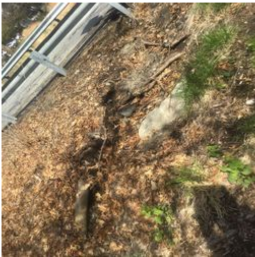
Roadside erosion conveyance into swale
