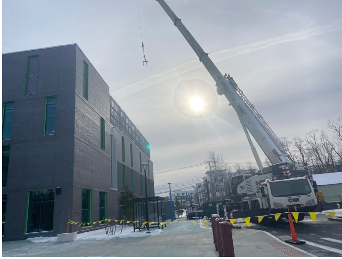
Solar Installation on Roof
